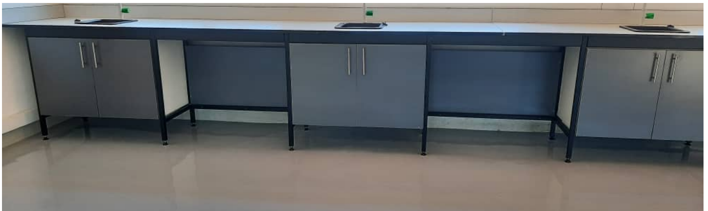
GUC MMOPANE WATER LABORATORY - TACHU INSTALLATION
